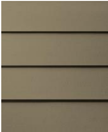
Fiber Cement Siding 2
