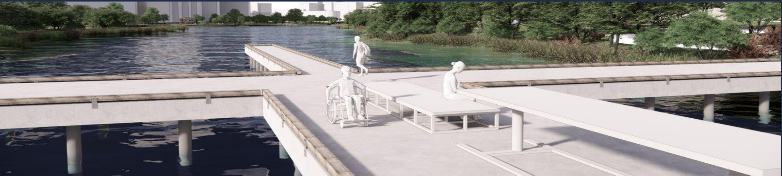
CASTING PIER IMPROVEMENTS
