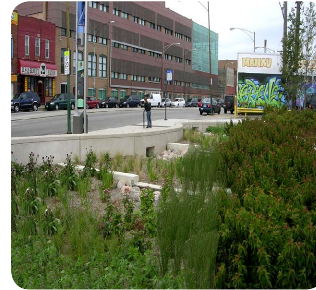
Figure 2: Stormwater street retrofit at Cermak/Blue Island
