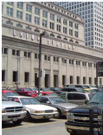
Image 2-20: The surface parking lot south of the station along Jackson is a prime site for an intermodal transfer facility.
