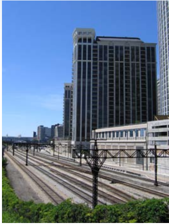
Image NS-4: The existing railscape south of Roosevelt will be improved visually.
