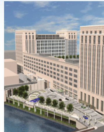
Image SW-4: Congress Parkway provides western access into the Central Area through the Old Post Office, which is proposed for mixed-use redevelopment as pictured.
