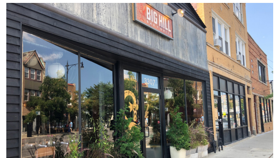
Contemporary and compatible new construction
