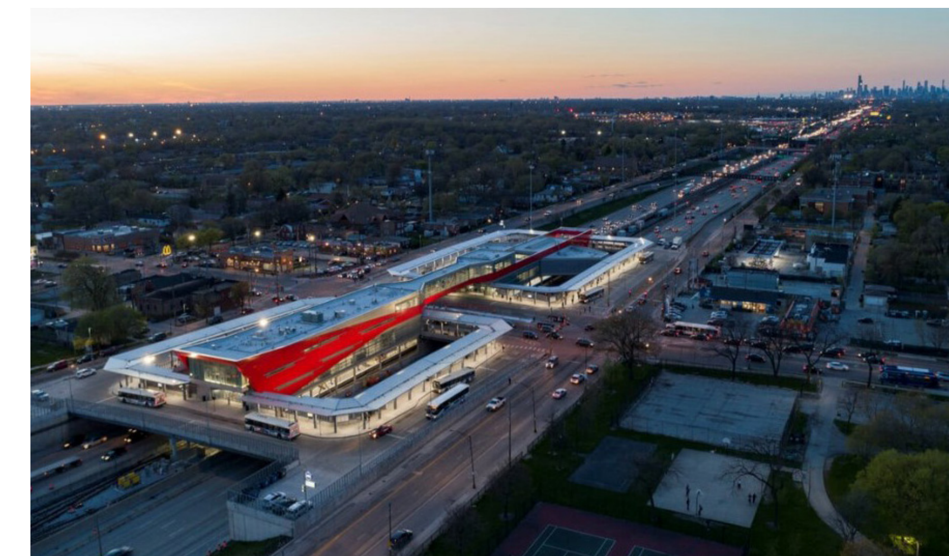
95th St Red Line Station
