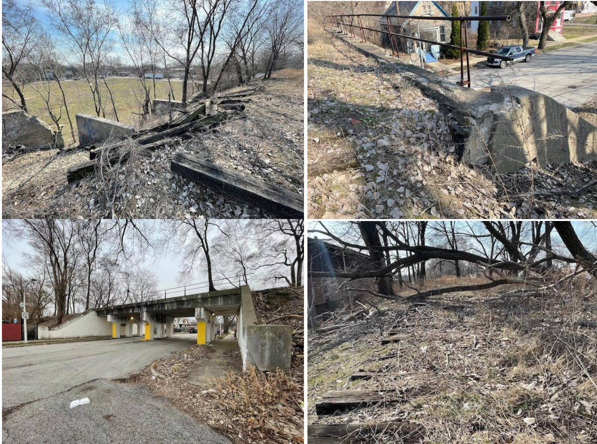
FIGURE 13. EXAMPLES OF EXISTING INFRASTRUCTURE ALONG THE ENGLEWOOD LINE TRAIL
