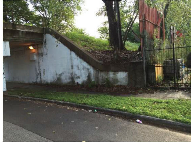
22 Green Street Viaduct
