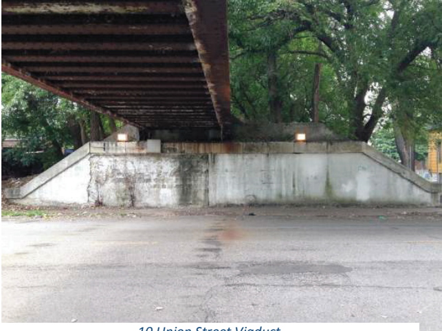
10 Union Street Viaduct
