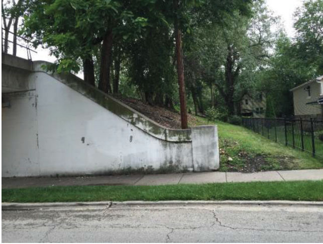
Morgan Street Viaduct
