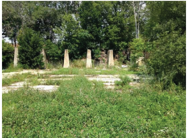
8 Emerald Avenue Auxiliary Structure
