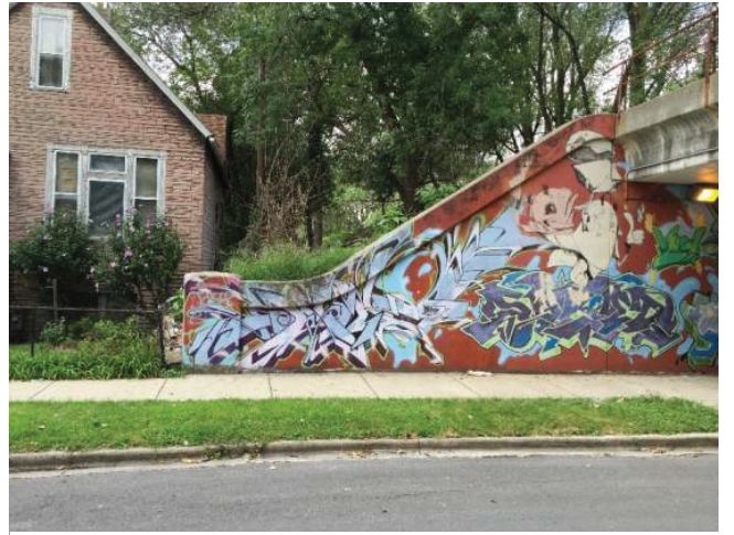
25 Carpenter Street Viaduct
