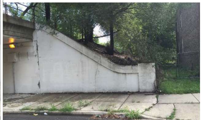
18 Sangamon Street Viaduct
