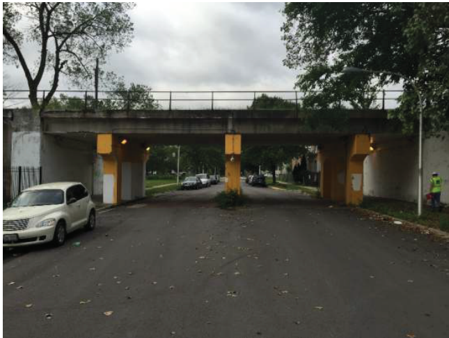
31 May Street Viaduct
