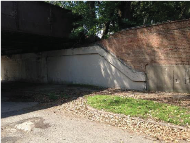
12 Emerald Avenue Viaduct
