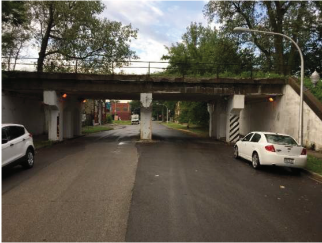
21 Green Street Viaduct
