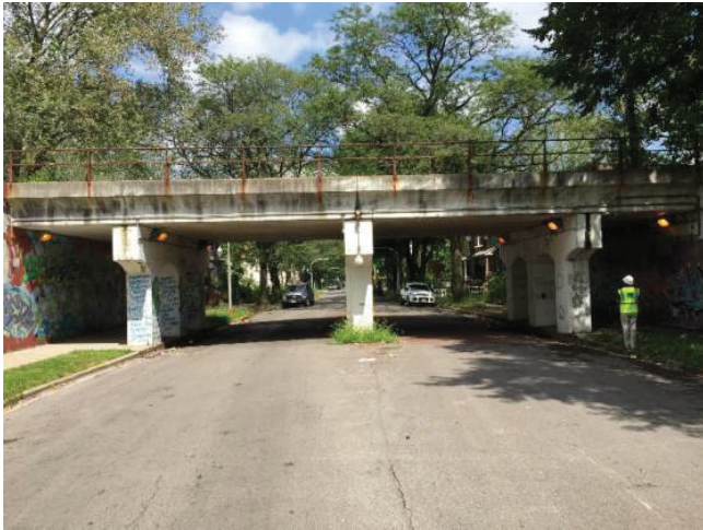
26 Carpenter Street Viaduct
