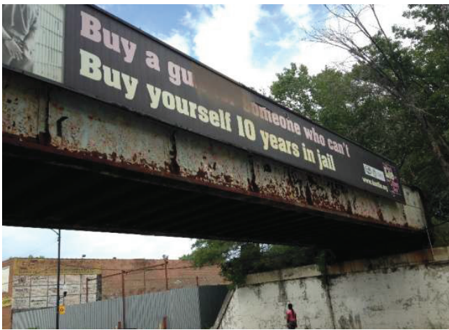
11 Halsted Street Viaduct
