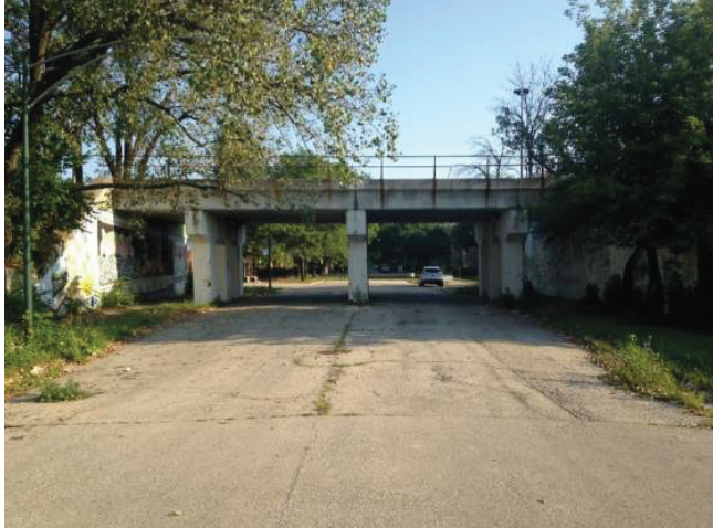
30 Elizabeth Street Viaduct
