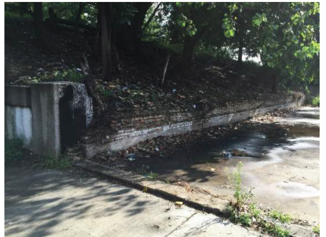
19 Peoria Street Viaduct
