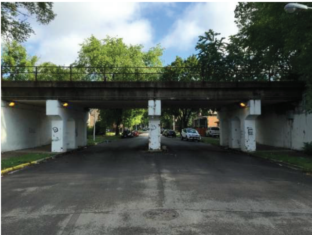
20 Peoria Street Viaduct
