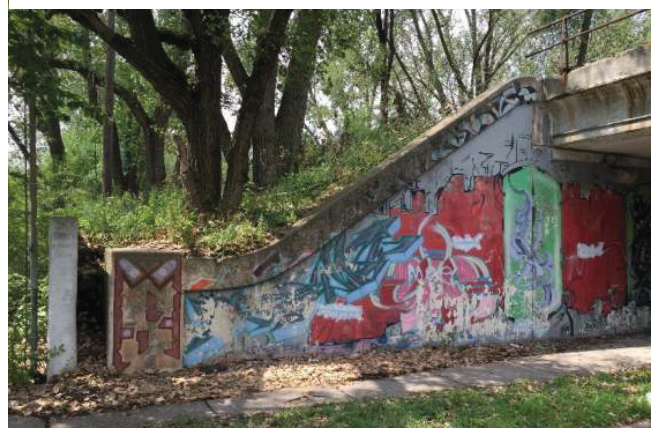
23 Aberdeen Street Viaduct
