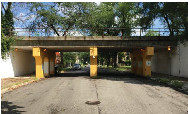
17 Sangamon Street Viaduct
