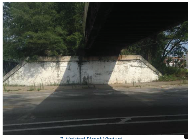
7 Halsted Street Viaduct
