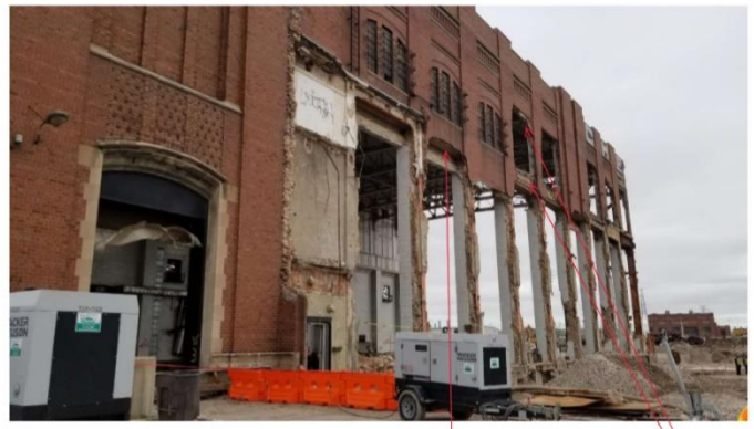
CRAWFORD POWER PLANT, SOUTH ELEVATION OF TURBINE BUILDING 5/4/20 BL01036
