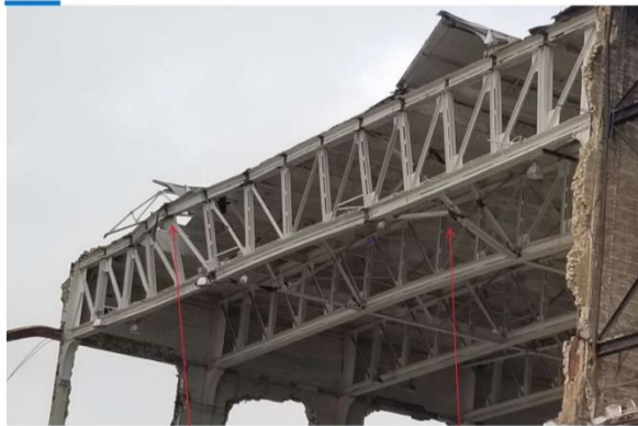
CRAWFORD POWER PLANT, EAST ELEVATION OF TURBINE BUILDING-ROOF TRUSS 5/4/20 BL01036
