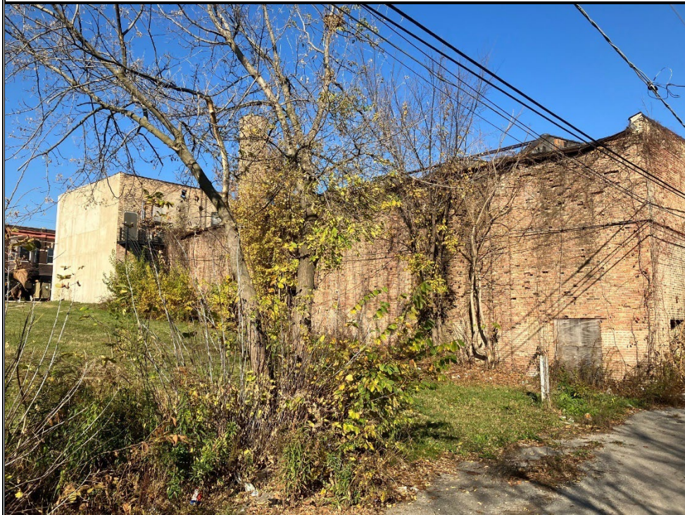
SUBJECT: LOOKING NORTHWEST
