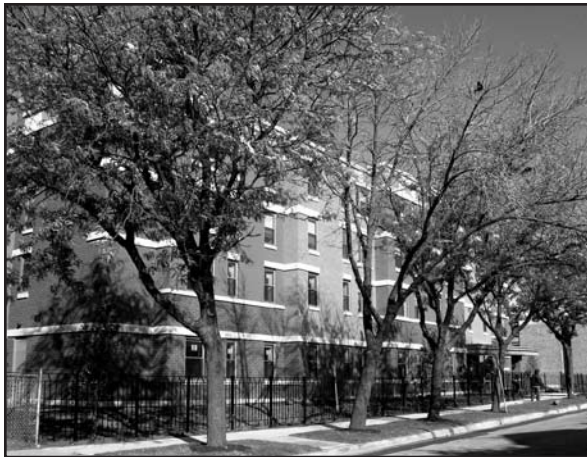
Coppin House, developed by Interfaith Housing Development Corp., has created 54 units of affordable rental housing for grandparents raising grandchildren as well as children "aging out" of foster care.
