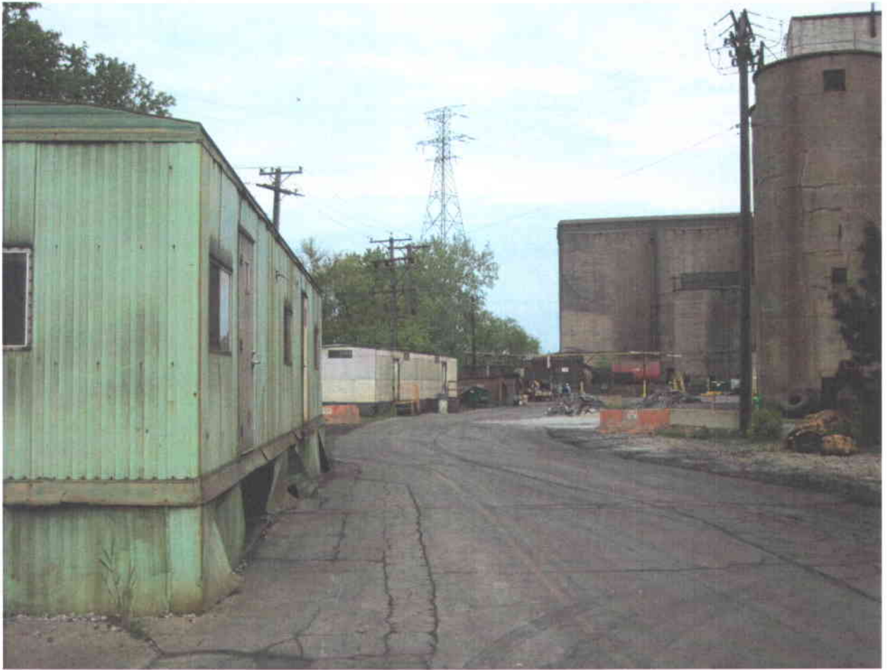
Test 12 – North Property Line (Downwind)
