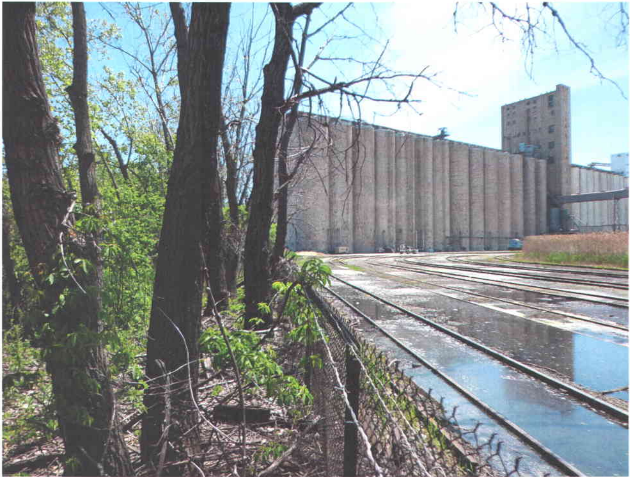
Test 13 – Property Line Segment D (Example Reading Location)
