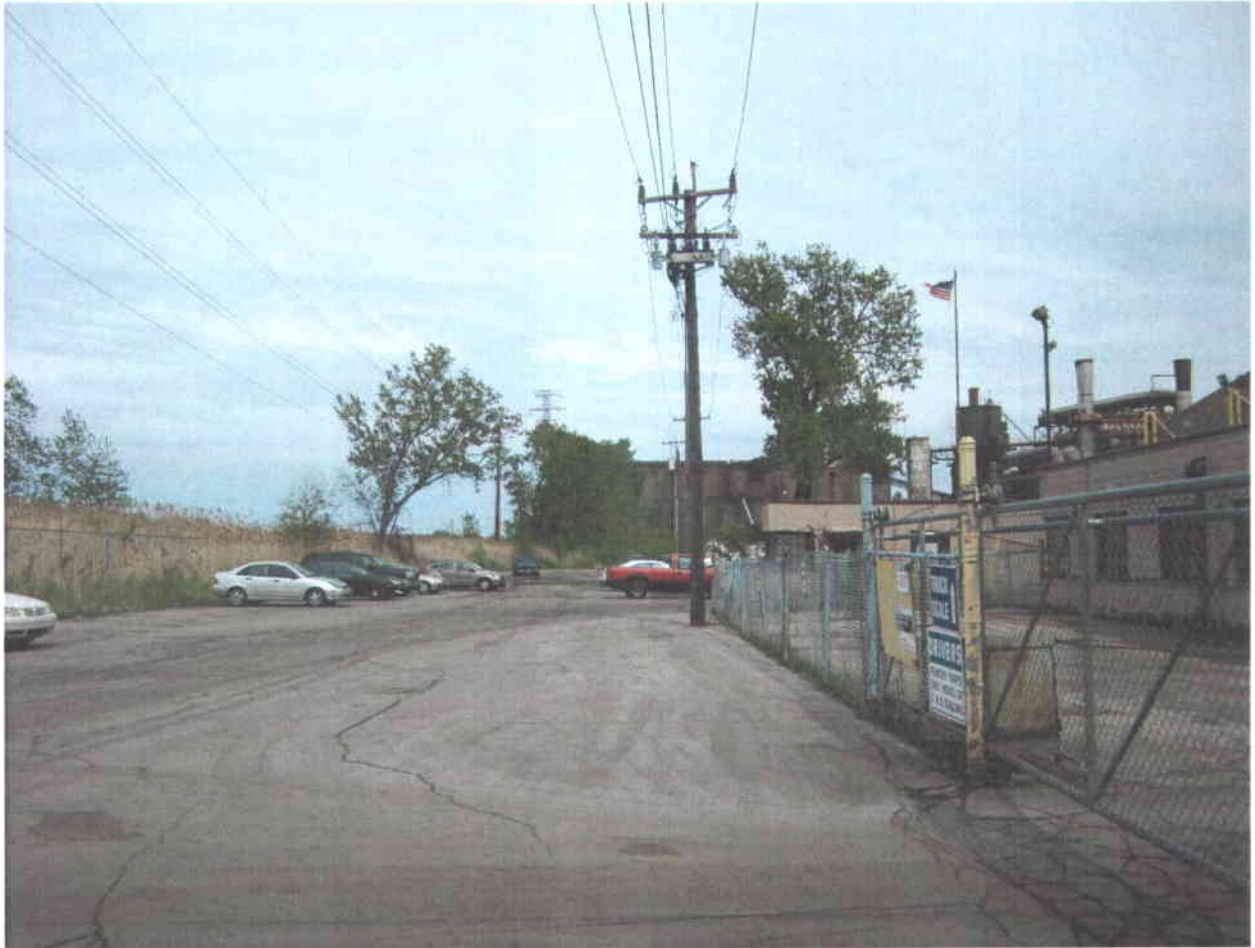
Test 13 – North Property Line, Segment 2
