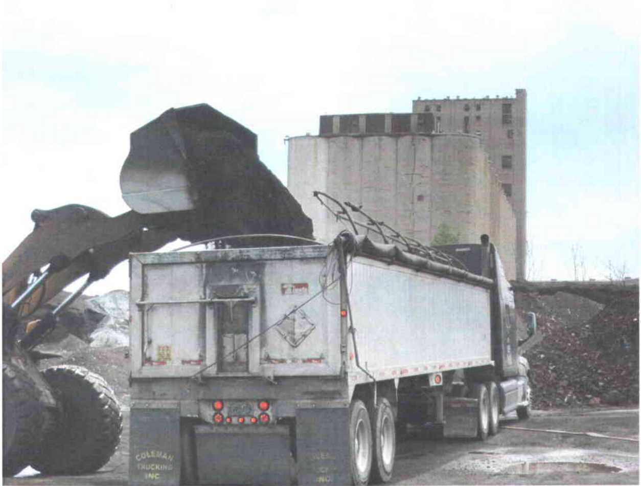
Test 14 – Temporary Stock Pile Truck Loading
