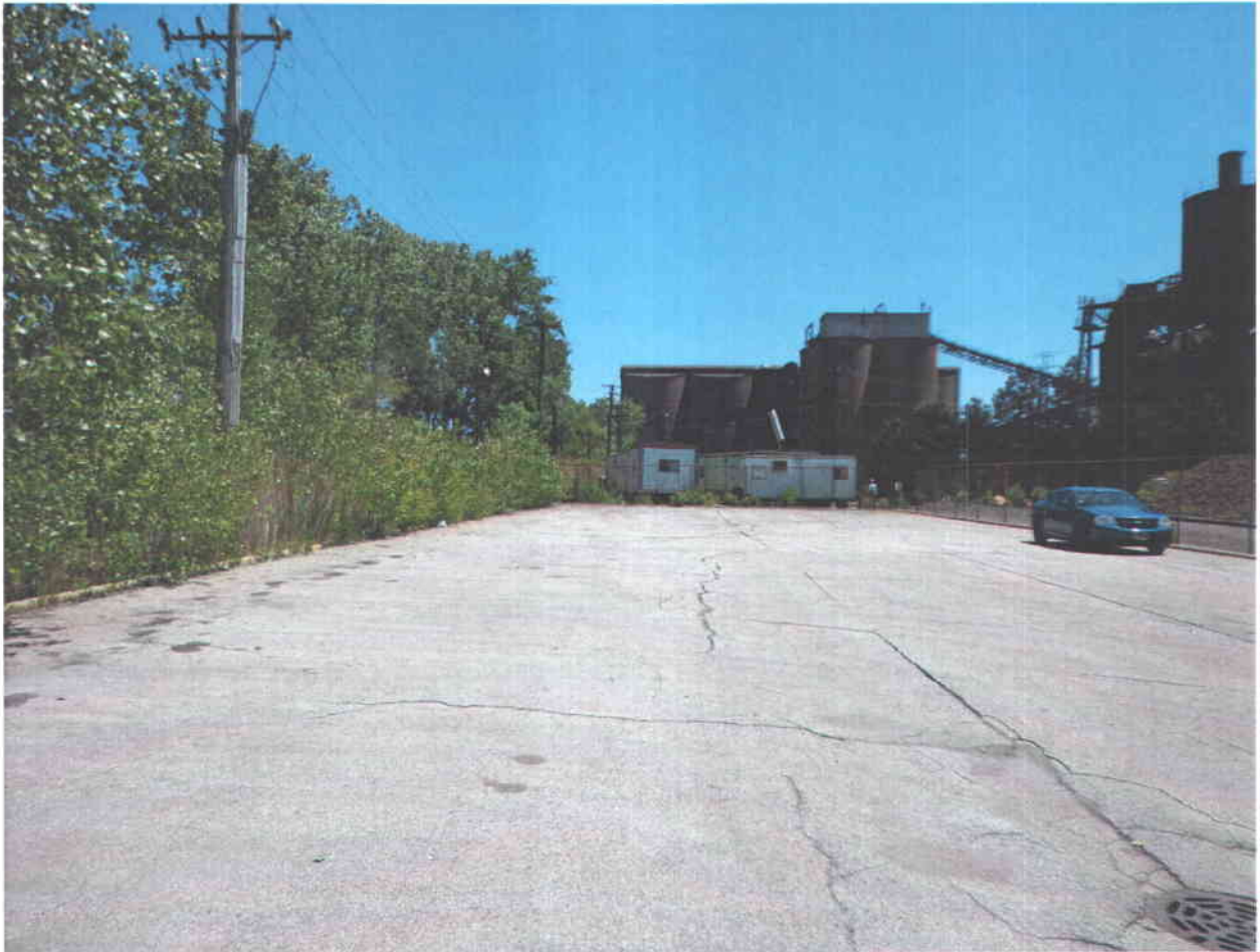
Test 13 – Property Line Segment G (Example Reading Location)
