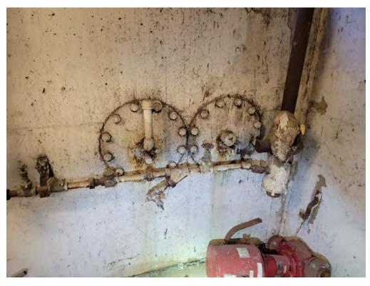
Suspect UST piping in boiler room.
