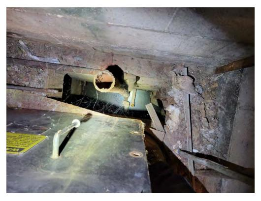
Suspect UST piping in boiler room.
