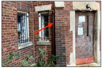
Suspect UST vent pipe located in northwestern portion of courtyard
