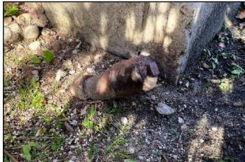
Suspect UST fill pipe located at northeastern portion of courtyard
