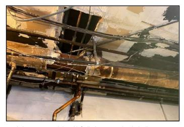
Asbestos containing AirCell pipe wrapping in boiler room
