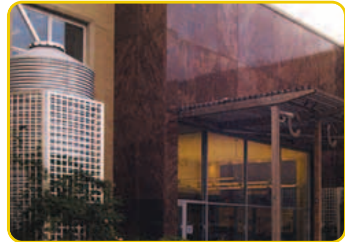
CCGT Site After
