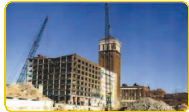
Sears Warehouse Construction Site
