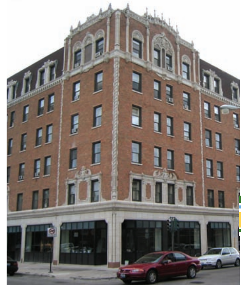
The Leland Apartments
