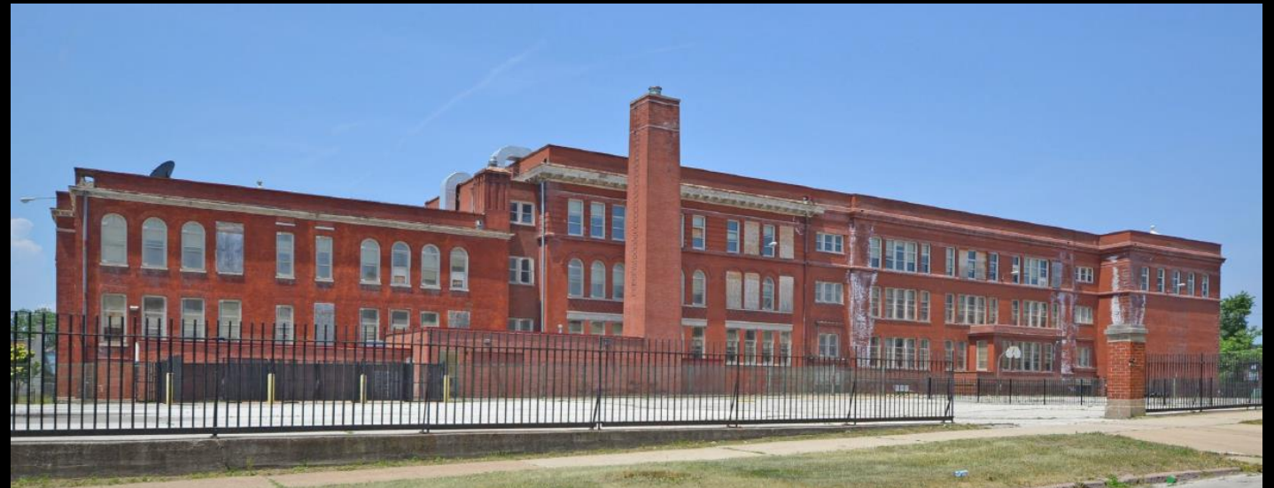
East Elevation & Boiler House Pre-Rehab
