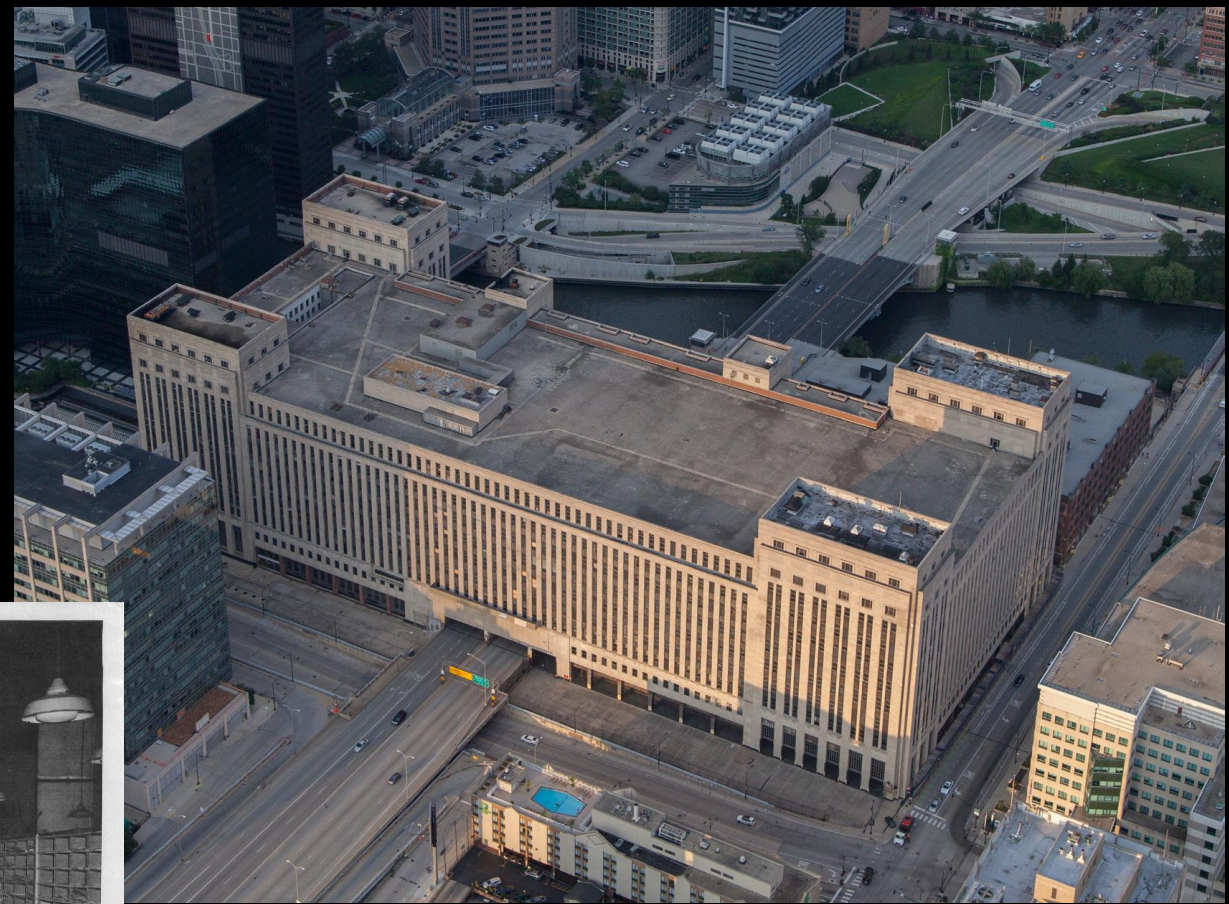
Roof and West Elevation, 2017
