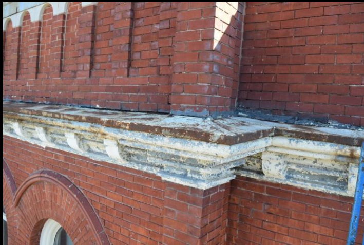
Metal Cornice Pre-Rehab
