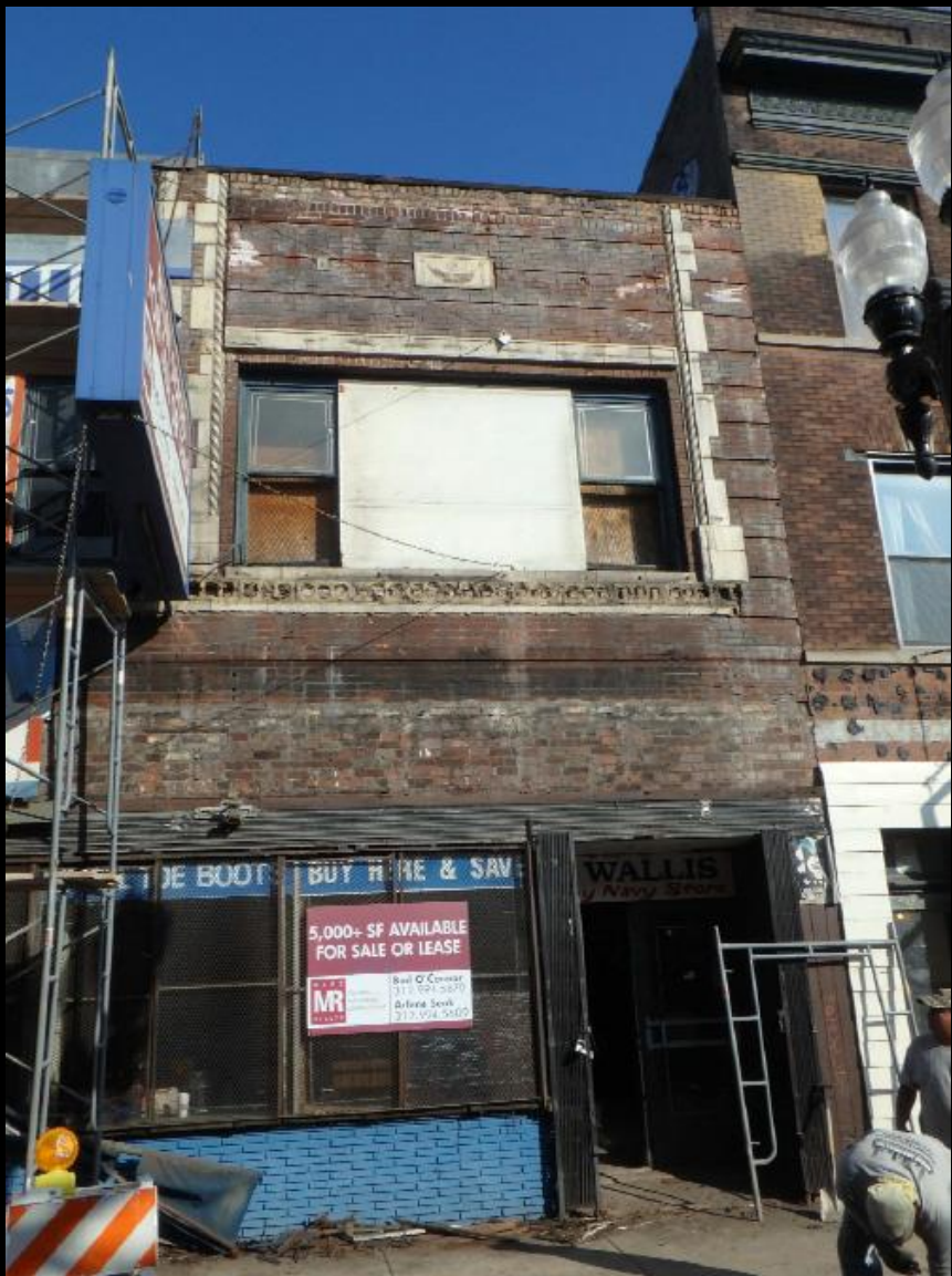
After Removal of Metal Panels
