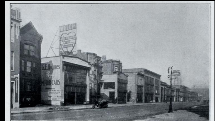
FIG. 1. AUTOMOBILE ROW. West Side, from 14th to 16th Streets, Michigan Boulevard, Chicago. Various Architects.
