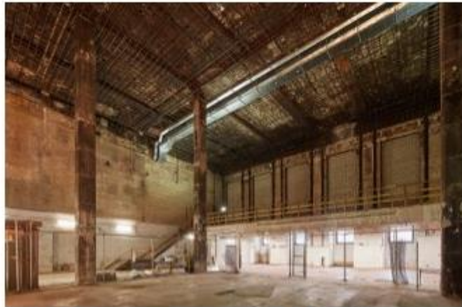
(10) PAST: View looking southwest towards South Clinton Avenue
