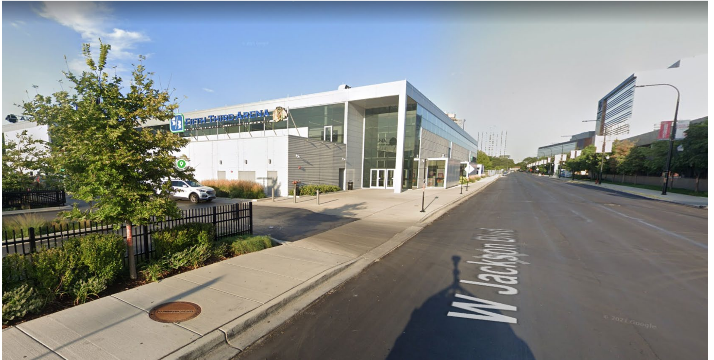
EXISTING CONDITIONS – JACKSON BLVD. at WOOD ST., LOOKING WEST
