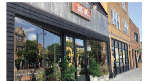
Contemporary and compatible new construction
