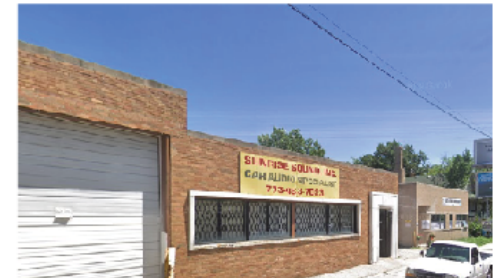
Kedzie, east side of street
